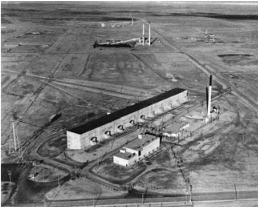
Completed chemical separation plants and steam-electric facility at Hanford, Wash.
