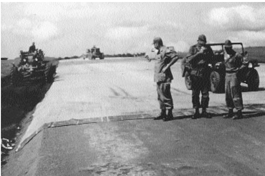
Installing T-17 membrane at Bao Loc
