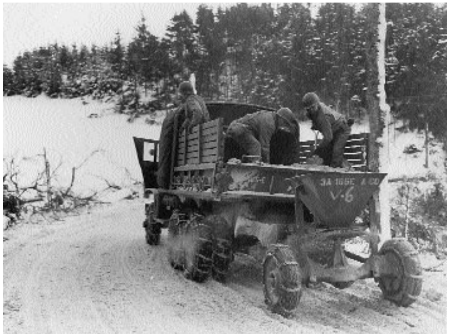
Army engineers sanding a road, Luxembourg, 1945
