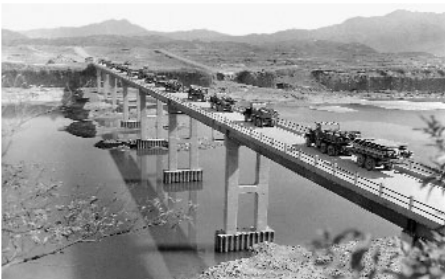
Built by the 84th Engineer Construction Battalion, the Libby Bridge provided a vital high-level crossing of the Imjin River, July 1953.
