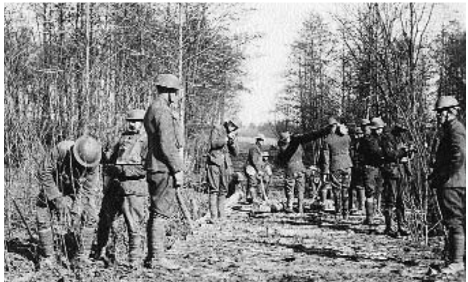
Engineers build a corduroy road
