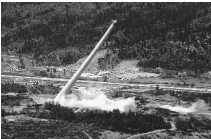
Demolition of a smokestack at a Bunker Hill, Idaho, Superfund site, 1995
