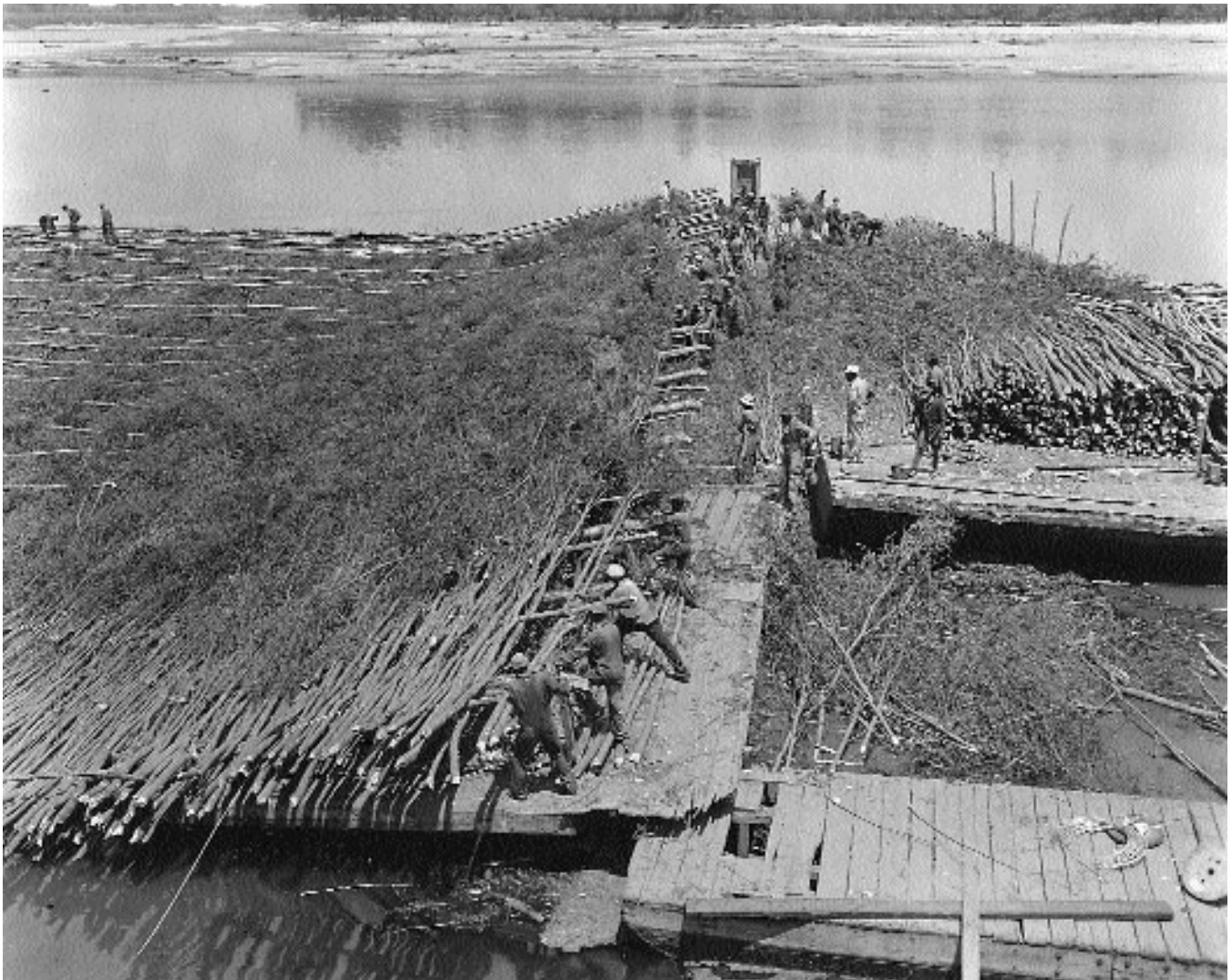
A willow mattress for bank protection along the Arkansas River, 1938
