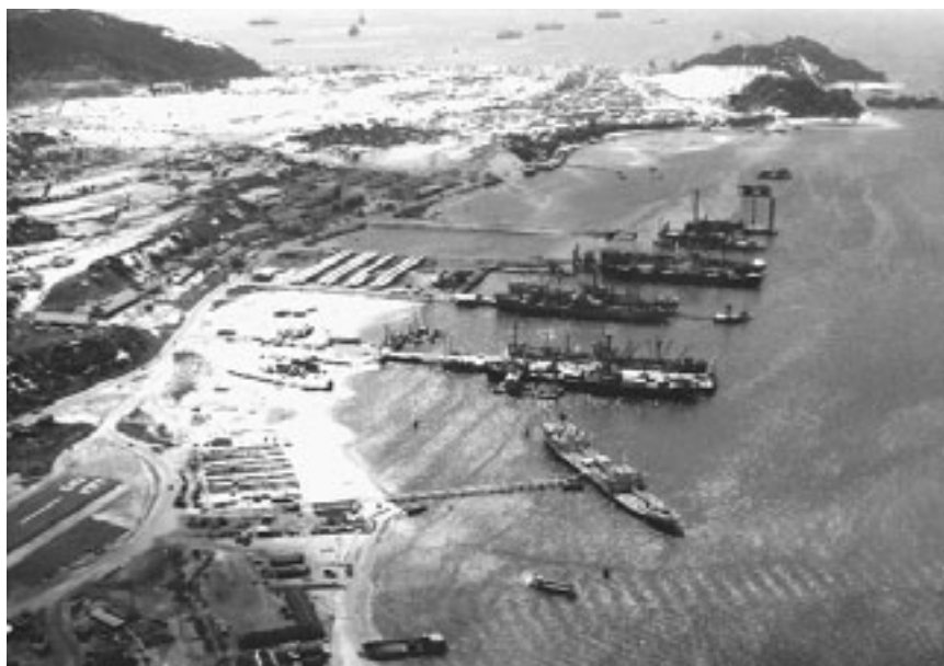
The port of Cam Ranh Bay showing newly constructed piers.
