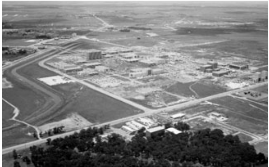
The Manned Spacecraft Center, Houston, Texas, under construction, December 1966.
