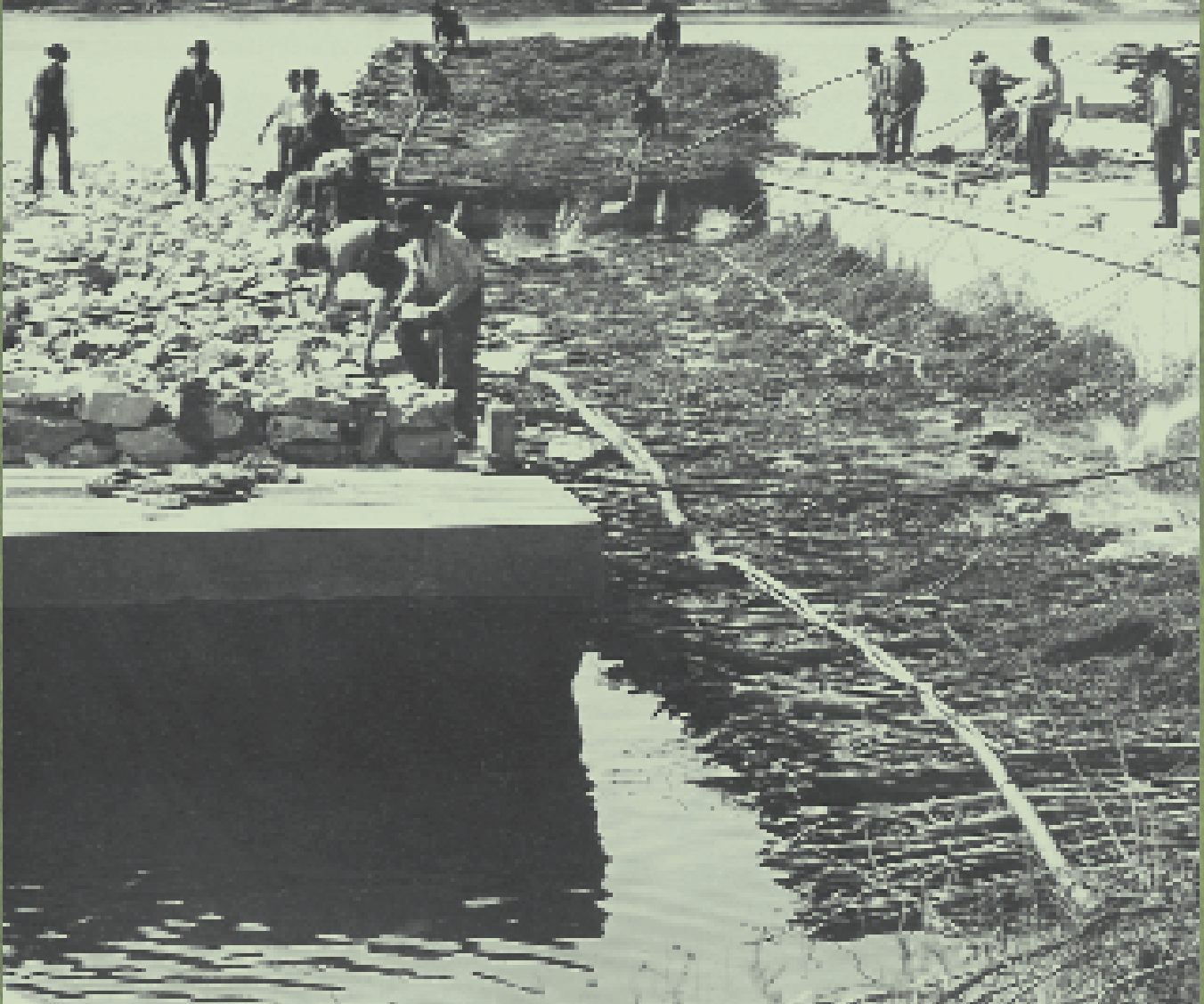
Construction of rock and brush wing dams on the Mississippi River in 1891. The photographer, Henry Peter Bosse (1844–1903), worked as a civilian engineer and draughtsman for the Corps of Engineers during the reshaping of the Mississippi River for modern transportation. Rediscovered only in the early 1990s, Bosse’s photographs have won international acclaim, earning him a place among the J. Paul Getty Museum’s “38 Photographers of Genius.”
