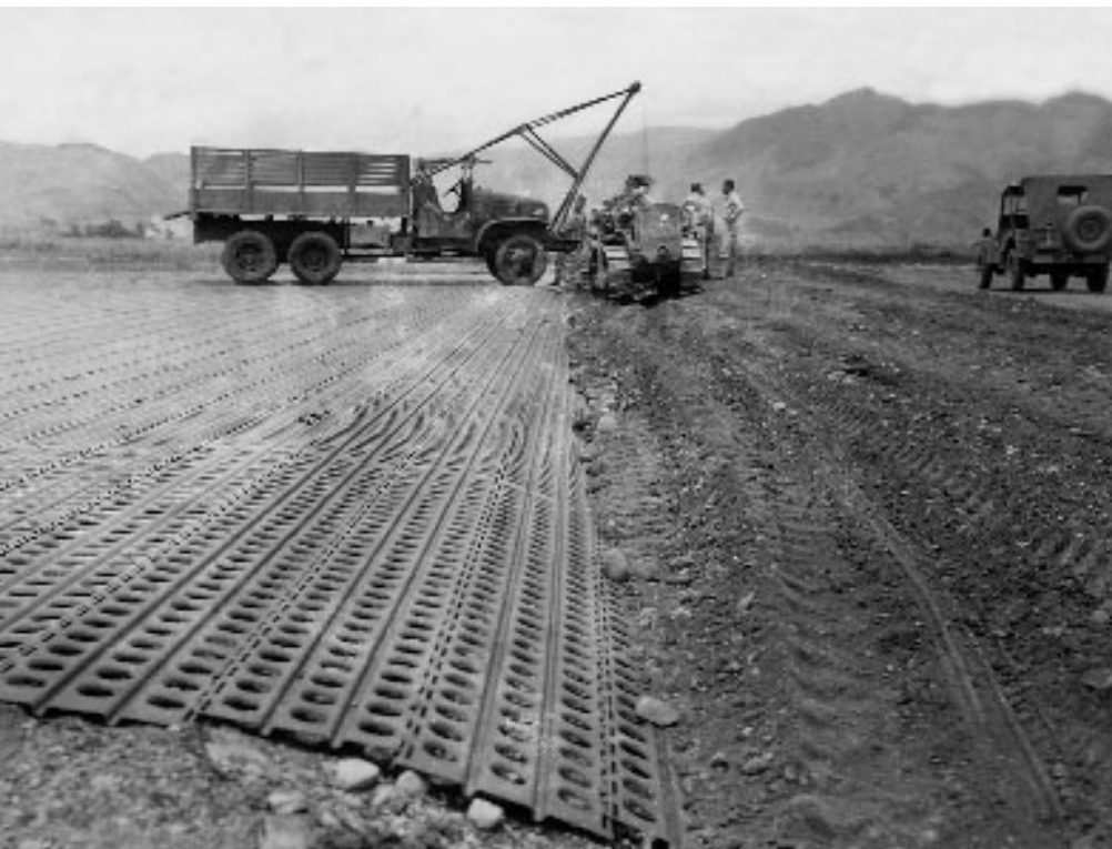
Engineers lay pierced-steel plank to construct a runway rapidly in New Guinea, February 1944
