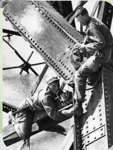
Engineers prepare a bridge for demolition in Korea National Archives
