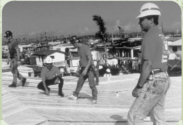
Installing temporary roofs following Hurricane Andrew
