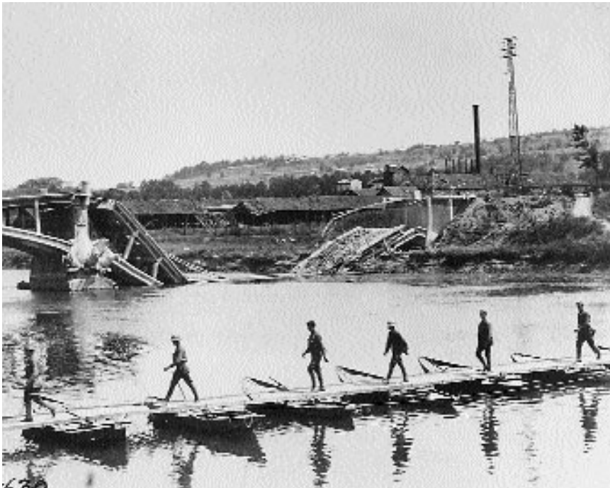
First ponton bridge over the Marne, July 20, 1918
