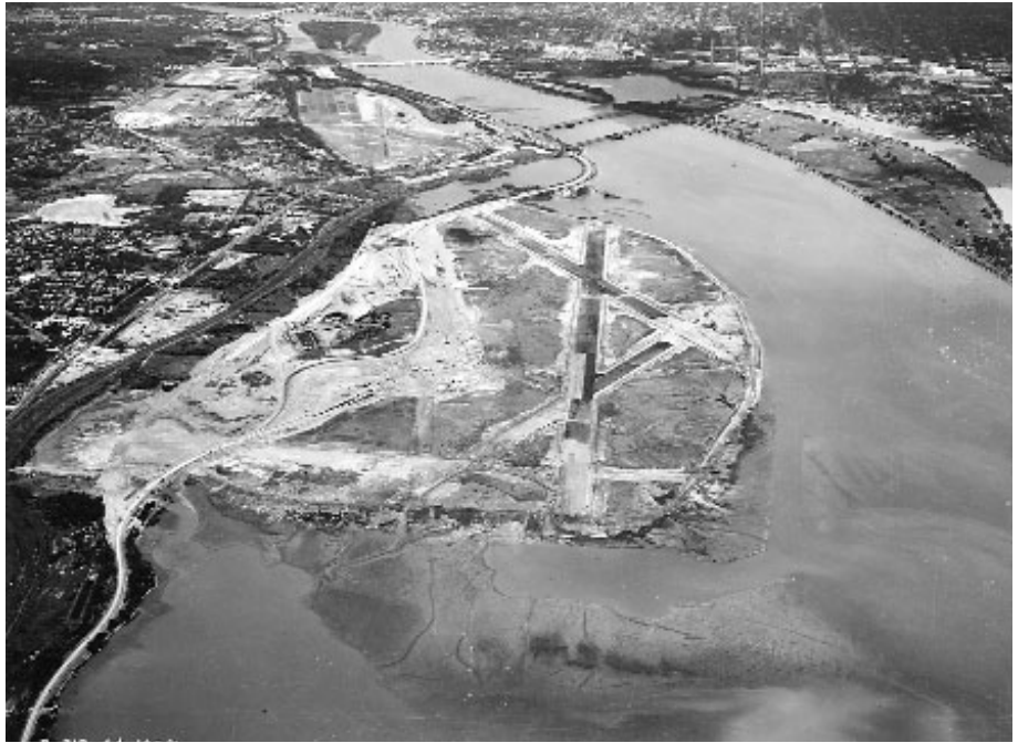
National Airport under construction, July 1, 1940
