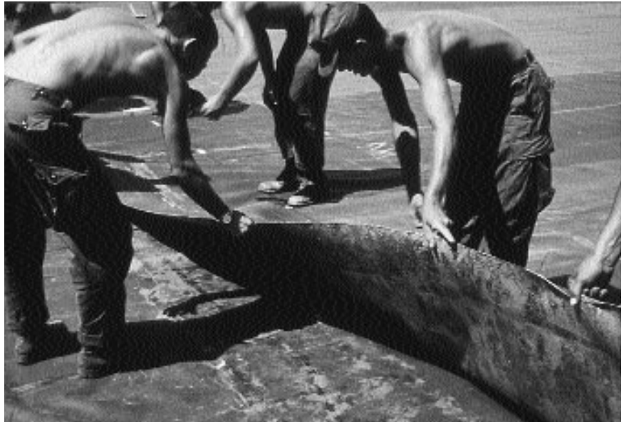
Spreading T-17 membrane on a runway
