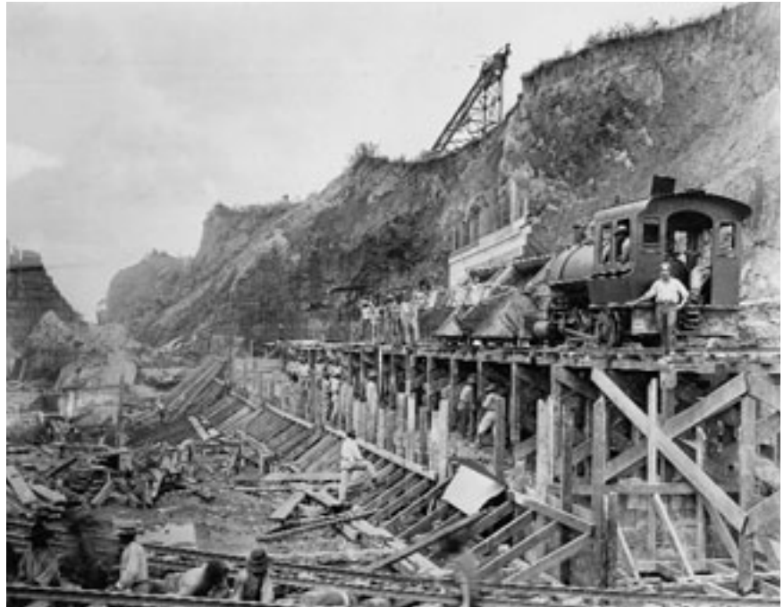
A rail line assisted the canal's construction.
