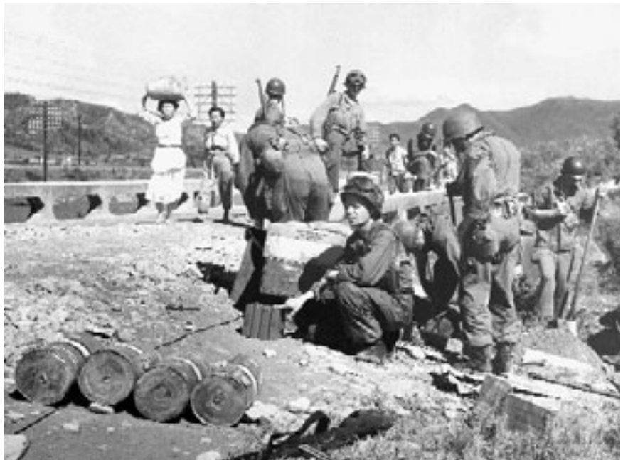
Engineers mine a bridge to impede the North Korean advance, July 1950 U.S. Army Engineer School
