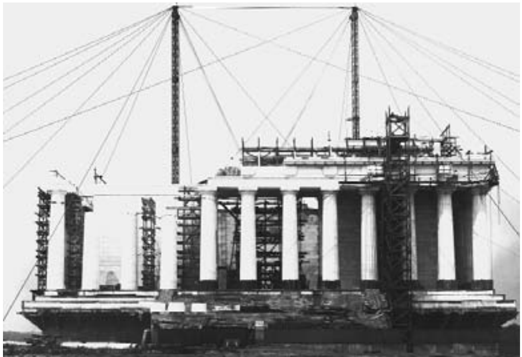
Lincoln Memorial under construction, July 1916
