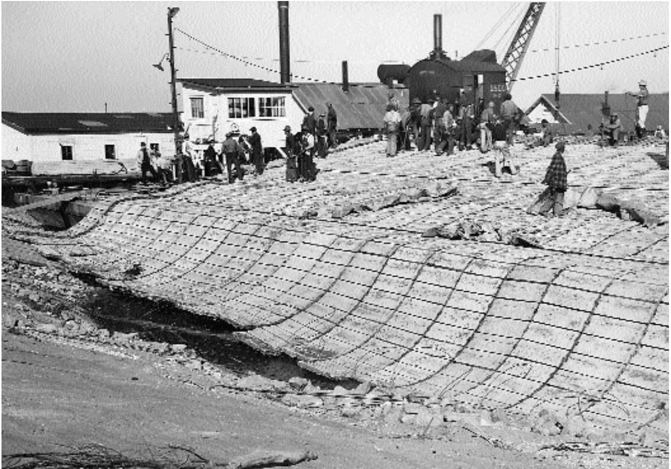
Barge and articulated concrete revetment along the Arkansas River, 1940
