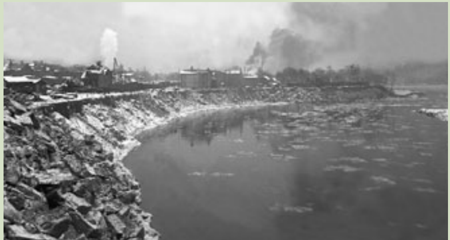
(above) View of eroded bank below abutment, Allegheny River, Dam 3, Jan. 1907
