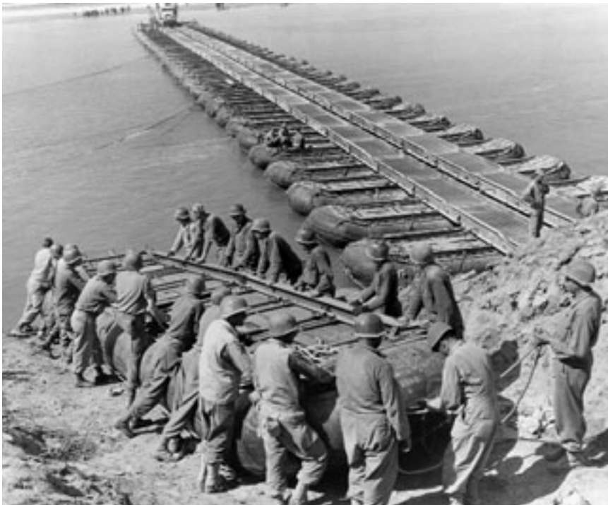
(below) Two 5th Army engineer units building a ponton bridge across the Po River north of Bologna, Italy, April 1945.
