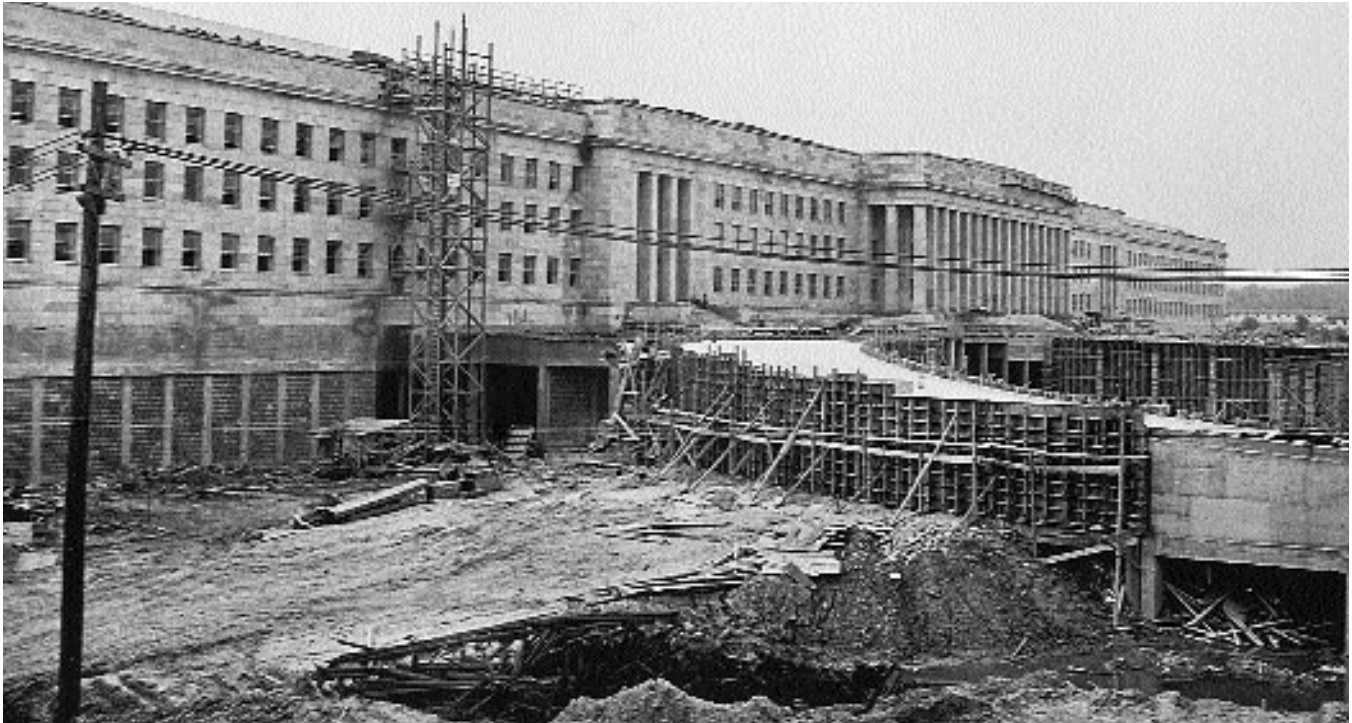
The Pentagon under construction
