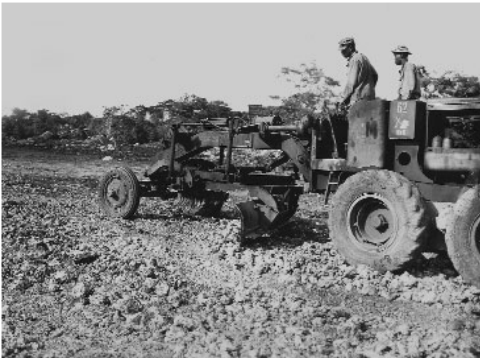
Engineers of the 856th Engineer Aviation Battalion, an African-American unit, grading an airfield on Kiriwina Island, east of New Guinea, October 1943.
