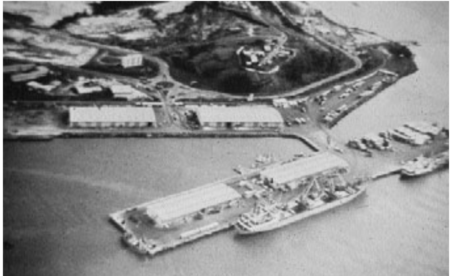
Port of Owendo, Gabon, site of Corps studies undertaken for the Agency for International Development
