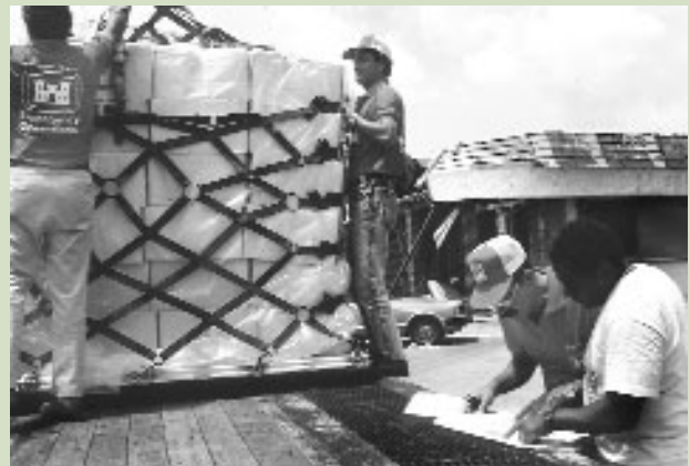
(right) Unloading roofing material, Cutler Ridge, Fla.
