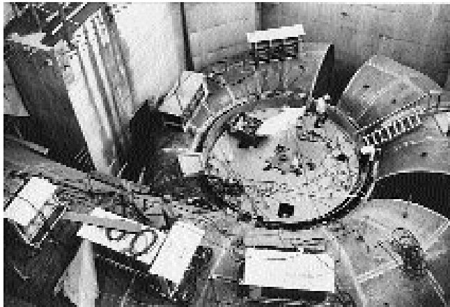
Powerhouse construction, Richard B. Russell Dam on the Savannah River, Ga., 1982
