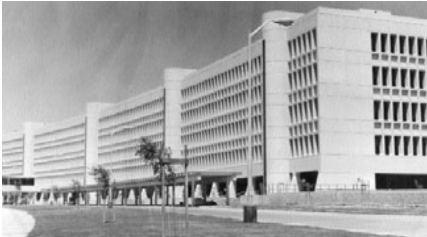
Saudi Arabian National Guard headquarters building
