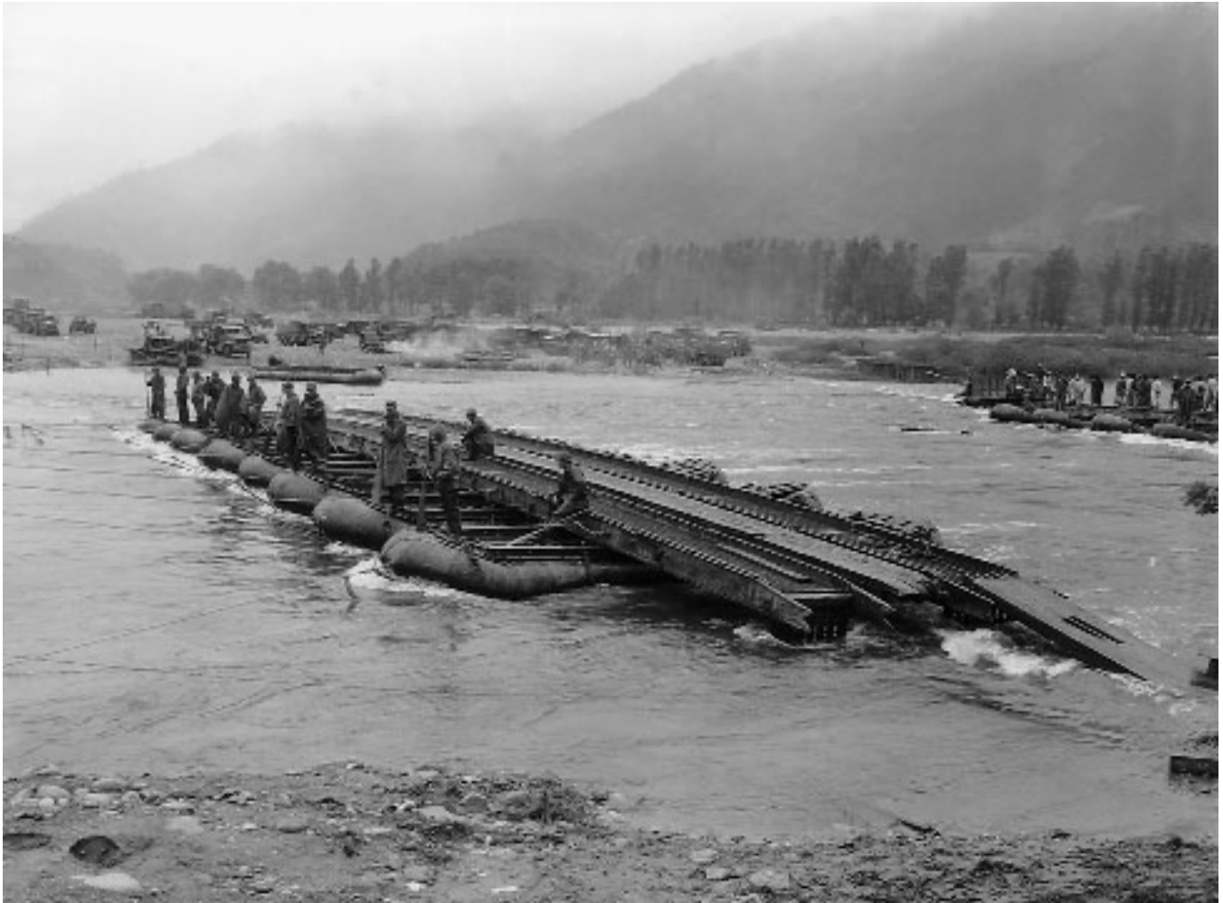
Soldiers of the 185th Engineer Combat Battalion stand watch over a floating bridge damaged by flood waters on the Soyang River, May 1951.
