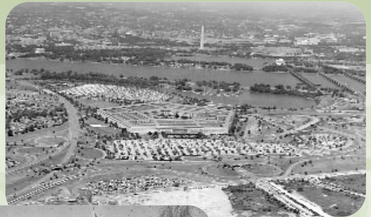
An aerial view of the completed Pentagon
