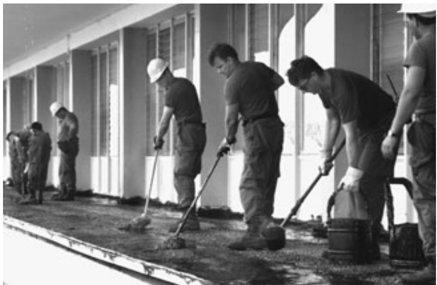
Military personnel repair the roof of a school damaged by Hurricane Andrew's strong winds.
