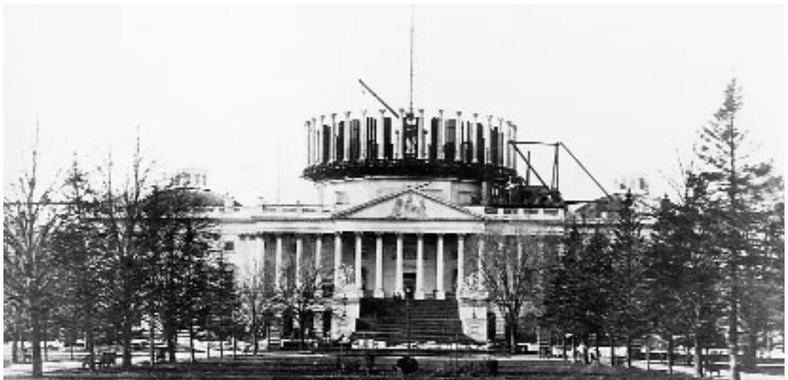
U.S. Capitol dome under construction, December 31, 1857
