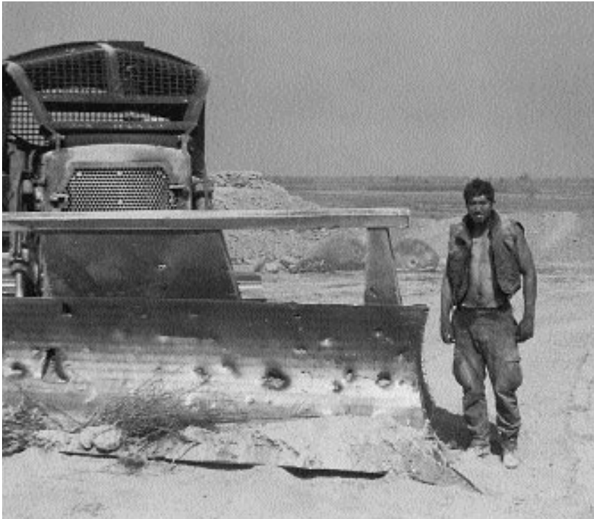
60th Land Clearing Company's Rome plow
