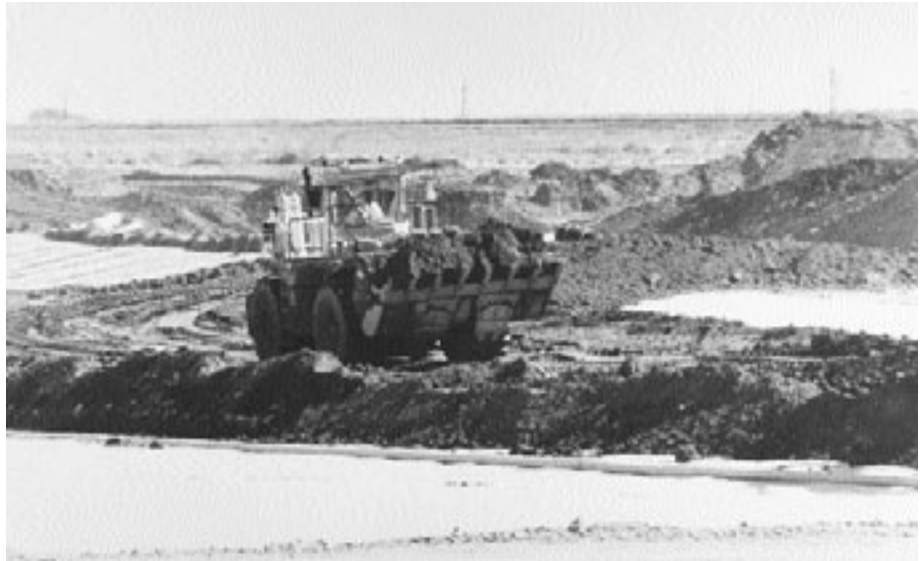
Removal of contaminated soil, Rocky Mountain Arsenal, near Denver, Colo.
