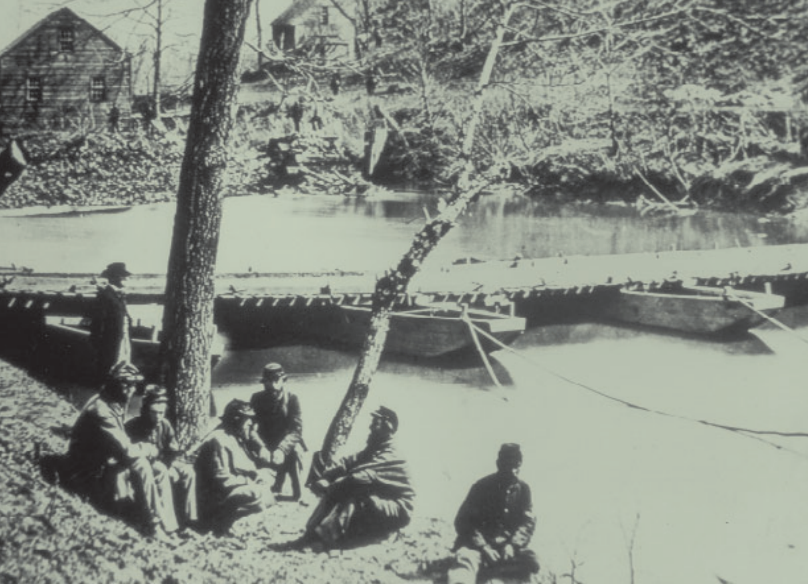
Civil War ponton bridge
