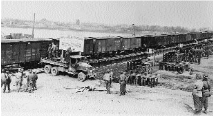
Gouldin railroad bridge on the Rhine built by Army engineers in ten days, April 1945
