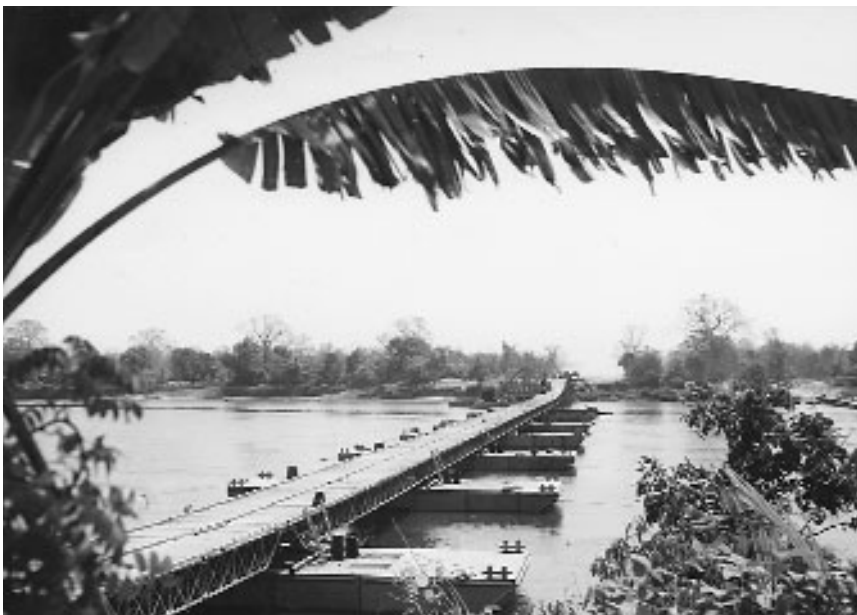
Steel barge bridge along the Ledo Road
