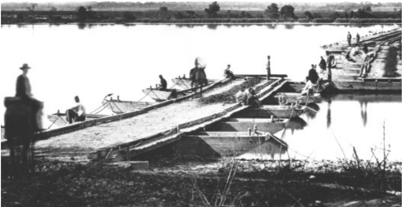
Ponton bridge under construction at Aiken's Landing on the James River, summer, 1864.
