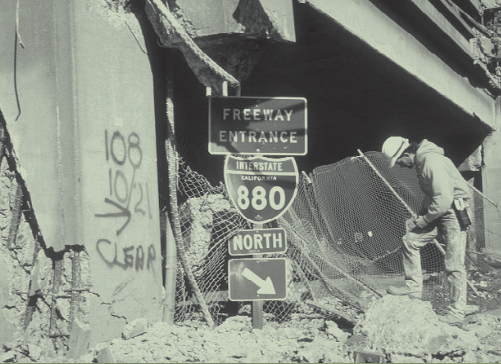
Damage assessment following the Loma Prieta earthquake, Oakland, Calif., October 1989
