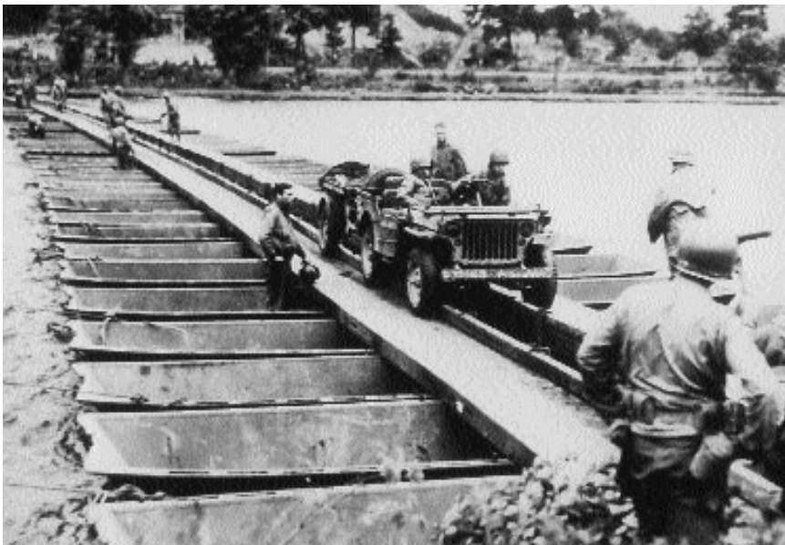
Crossing the Seine on a ponton bridge, August 1944
