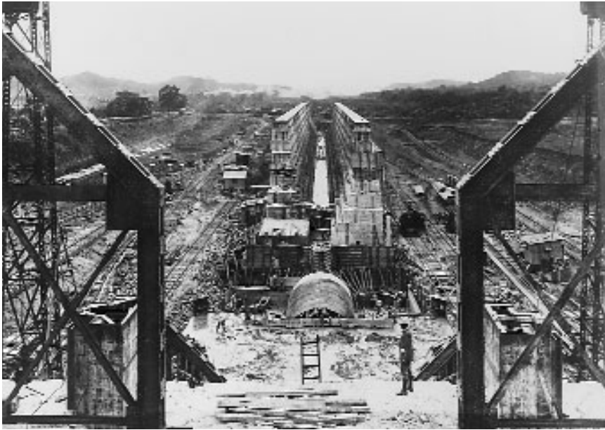
Construction of Pedro Miguel Lock, 1911
