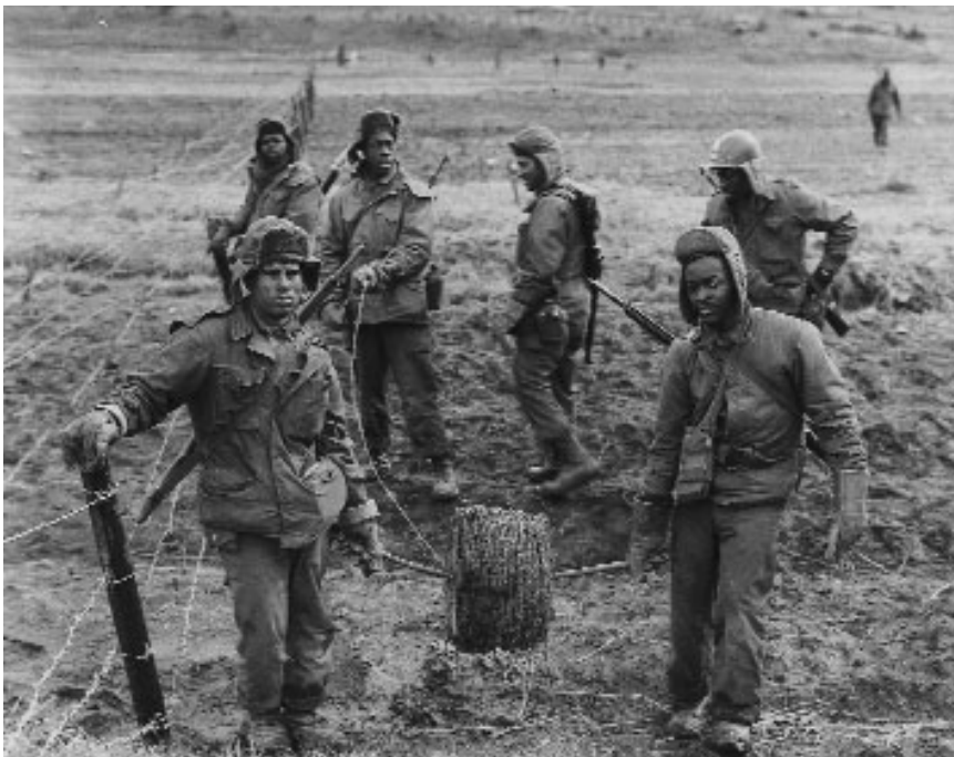
Soldiers of the 77th Engineer Combat Company lay a single-apron barbed wire fence National Archives
