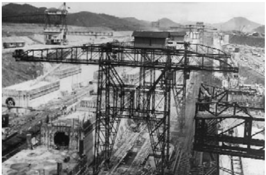
Miraflores Locks under construction, August 1912
