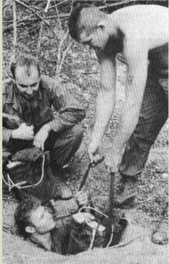
An engineer tunnel demolition team Department of Defense
