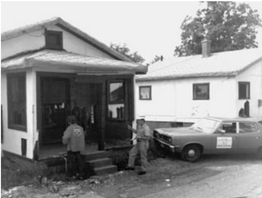
A Corps of Engineers disaster survey team inspects damaged homes following Tropical Storm Agnes.
