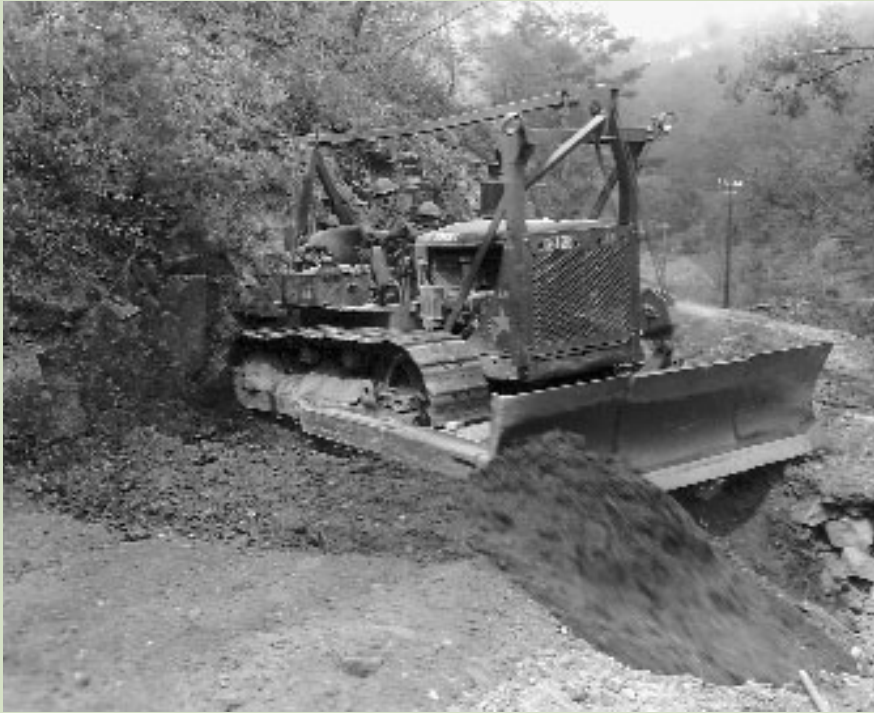
An engineer uses a bulldozer to repair a road damaged by retreating enemy troops. National Archives
