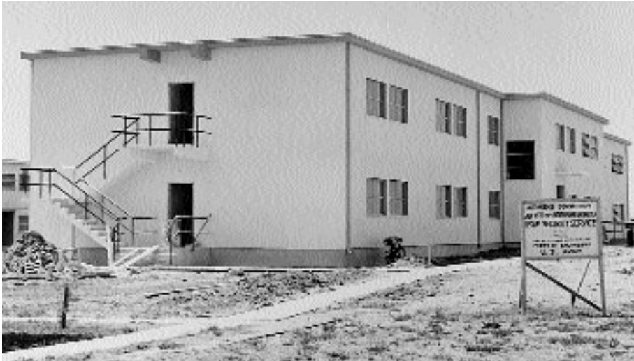
Air Force Dormitory, Brindisi, Italy, 1965
