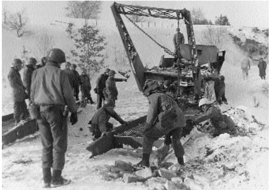
Assembling a treadway bridge in Belgium, 1945
