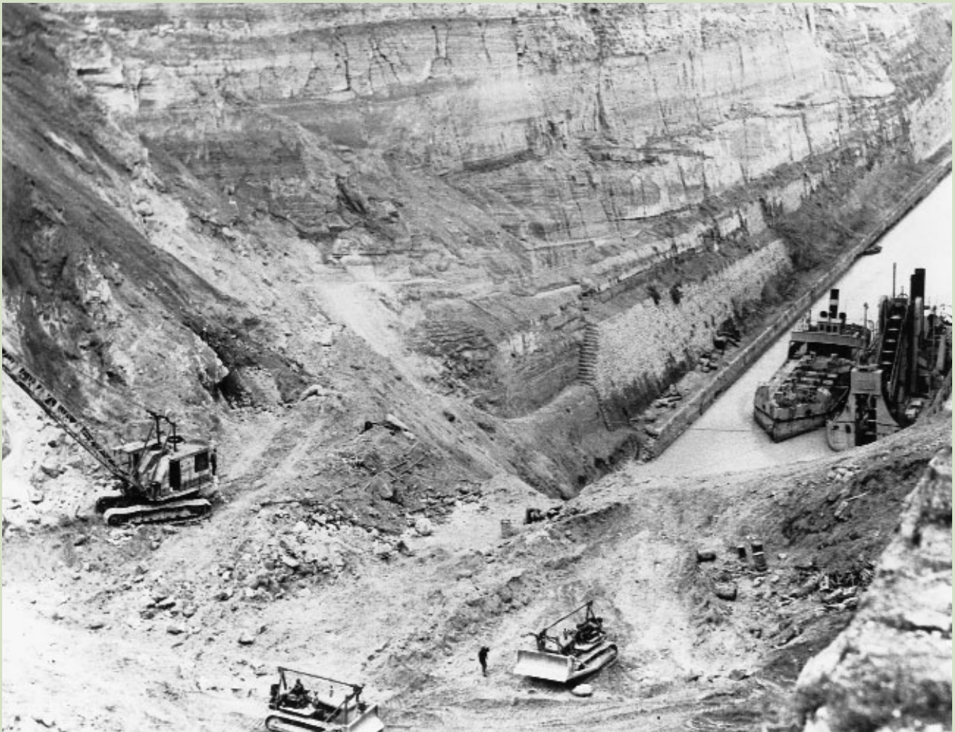
The dredge Poseidon clearing the Corinth Canal, 1947
