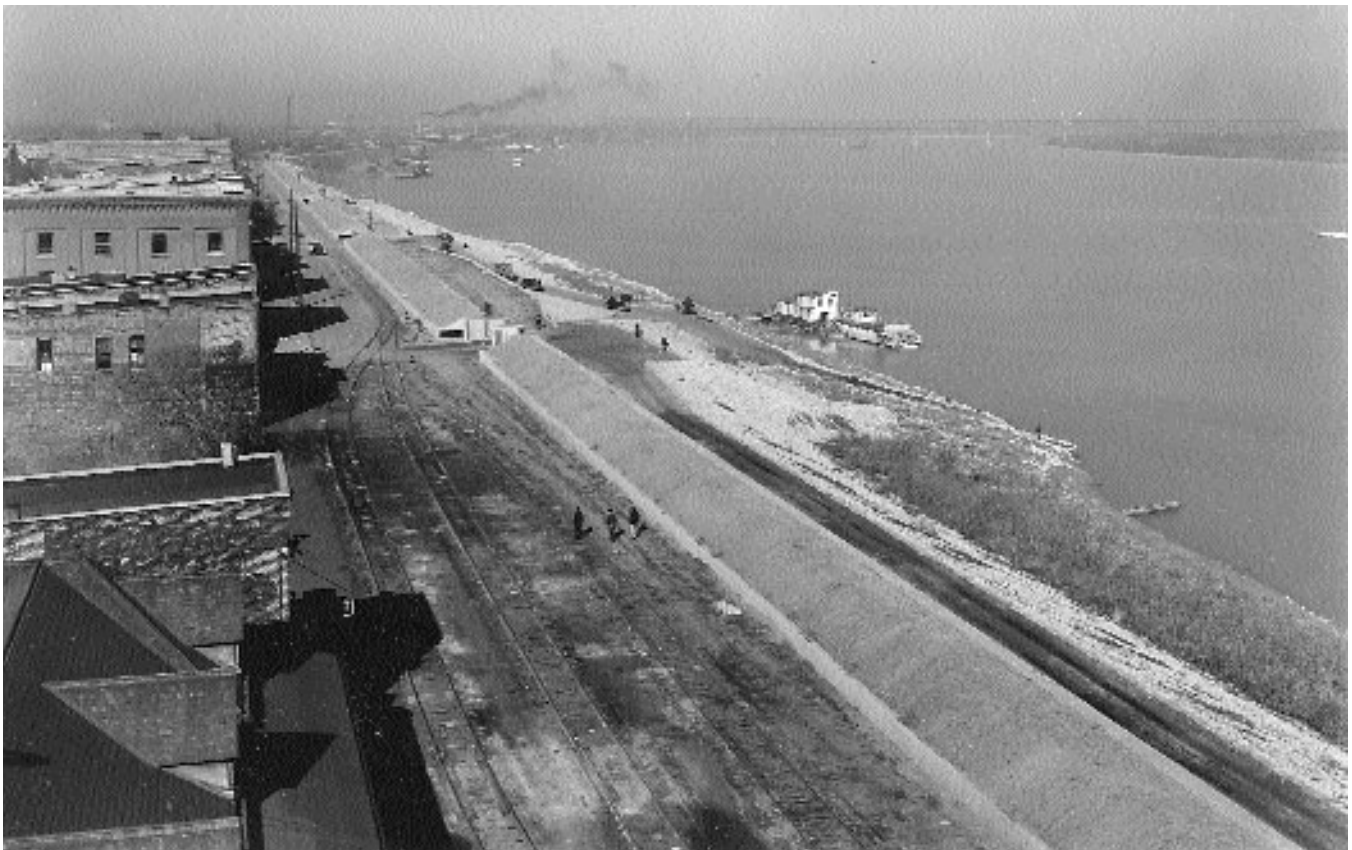
Floodwall at Cairo, Ill., 1936
