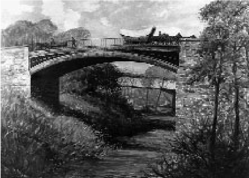
First cast-iron arch bridge built in the United States. Carl Rakeman painted this image of the Dunlap Creek Bridge.
