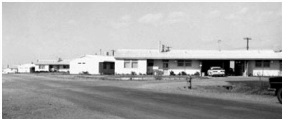
Family housing constructed at Ben Guerir, Morocco, in the late 1950s as the Corps built airfields to allow Air Force heavy bombers to reach the Soviet Union.
