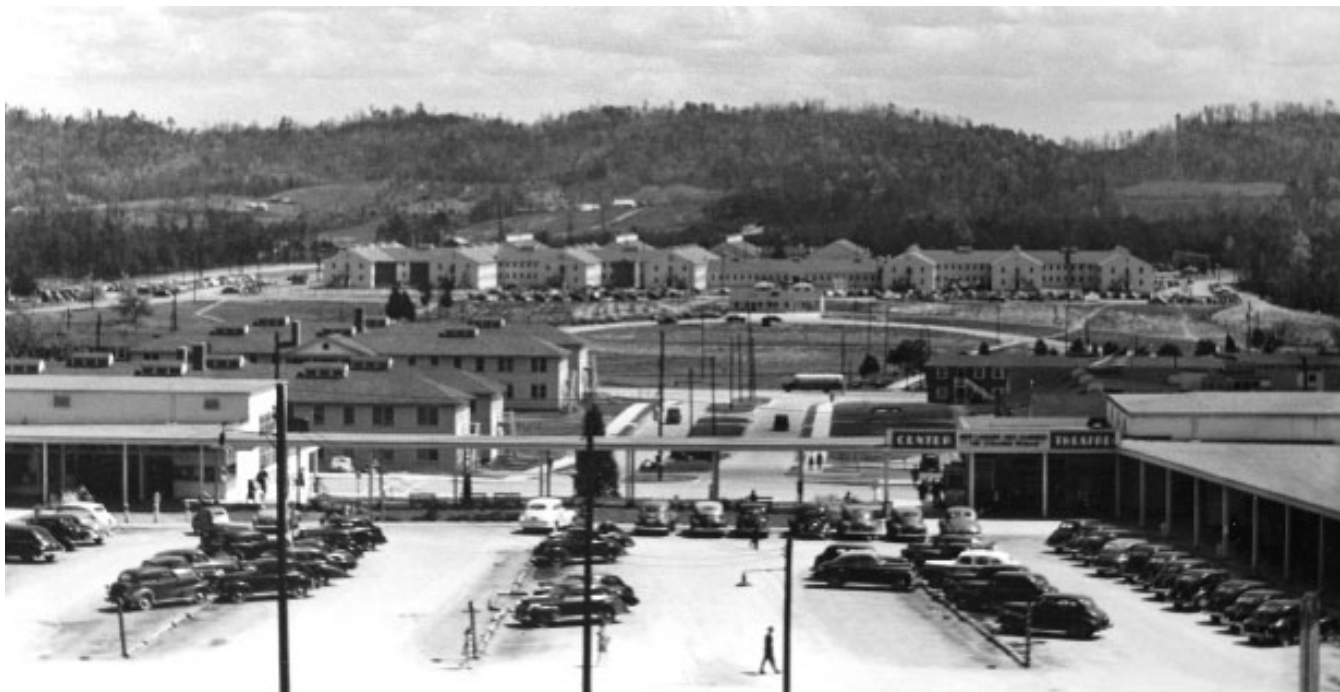
Oak Ridge, Tenn., shopping center (foreground) and district headquarters (background)
