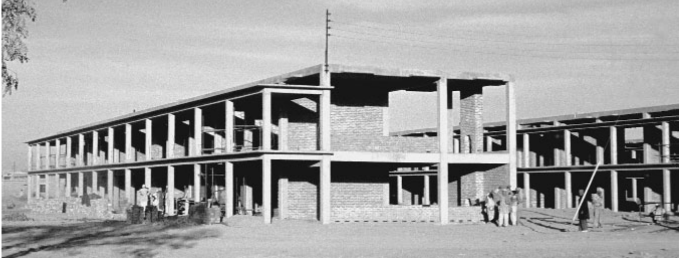
The Corps built a cantonment for the Pakistani army at Multan to accommodate 8,500 troops. The barracks above were two structures of the 310 built on the post. Construction at Multan began in 1959 and was complete two years later.
