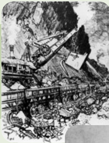
Steam shovel at work in the Culebra Cut; a lithograph in a series on the Panama Canal by Joseph Pennell, noted American artist and illustrator
