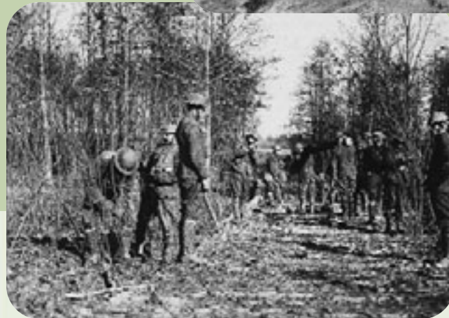
World War I Army engineers building a corduroy road
