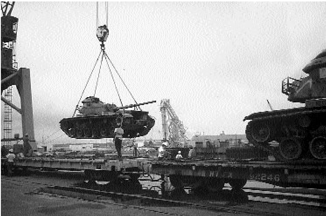
"Tanks to Reef" Project in Mobile District: The Corps used surplus tanks to help create a 1,000-square-mile artificial reef zone near Mobile, Ala., 1994.
