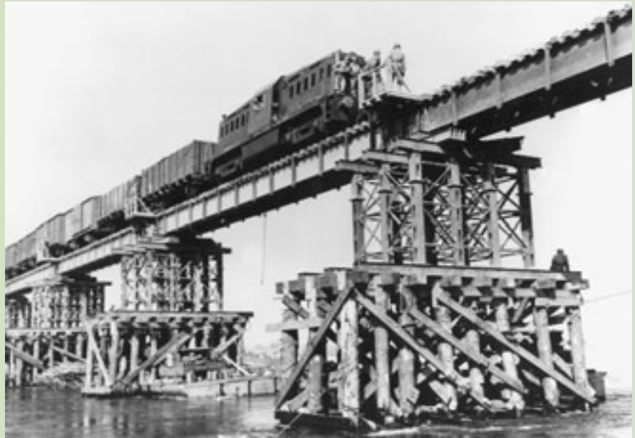
Railroad bridge over the Rhine built by Army engineers, April 1945
