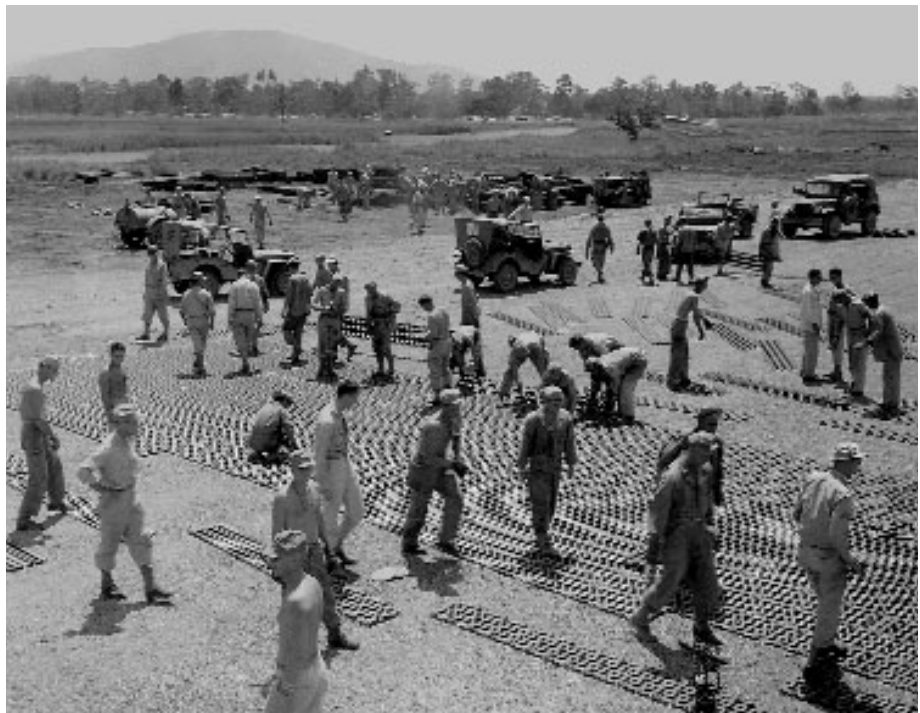
Laying pierced-steel plank on an airstrip at Nadzab, New Guinea, February 1944.
