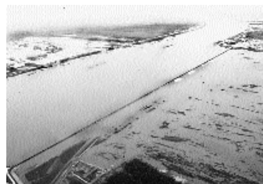
Floodwater over Bonnet Carré Spillway
