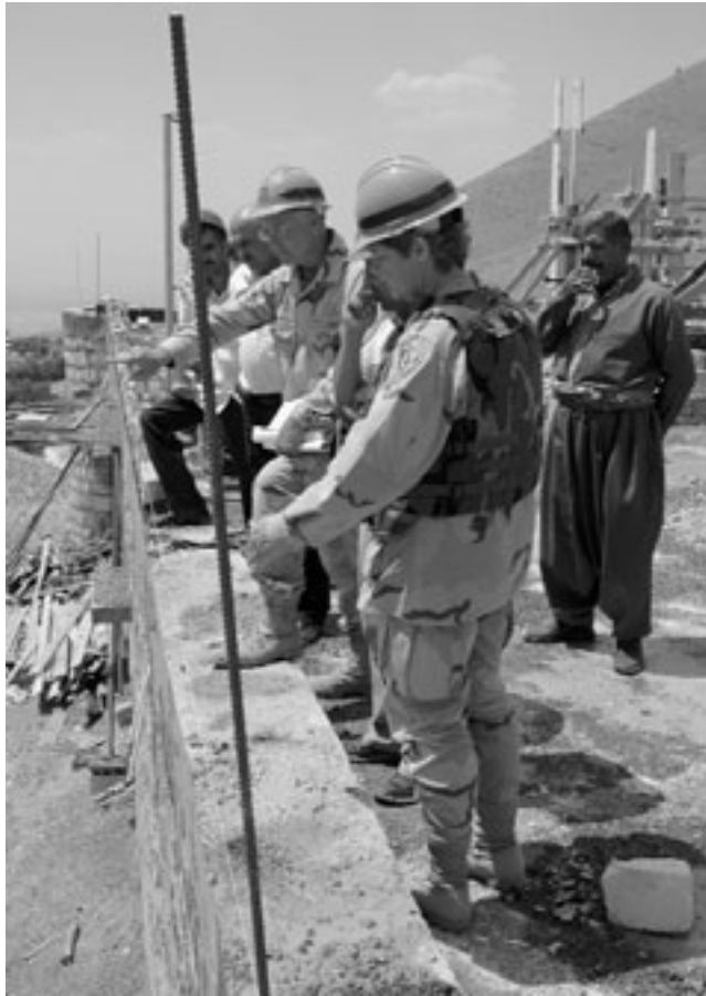
Engineers inspect the construction of a border fort near Kirkuk, May 2005.
