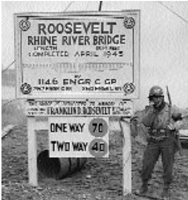
Roosevelt Bridge over the Rhine
