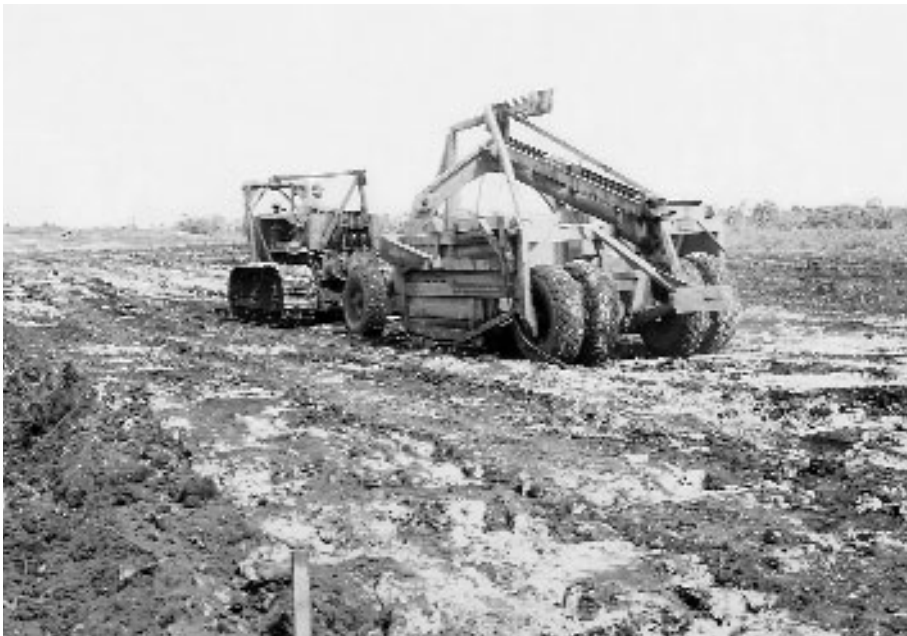
Engineer aviation battalions used heavy equipment such as bulldozers and carryalls to construct airfields for heavy bombers, Kiriwina Island, July 1943.
