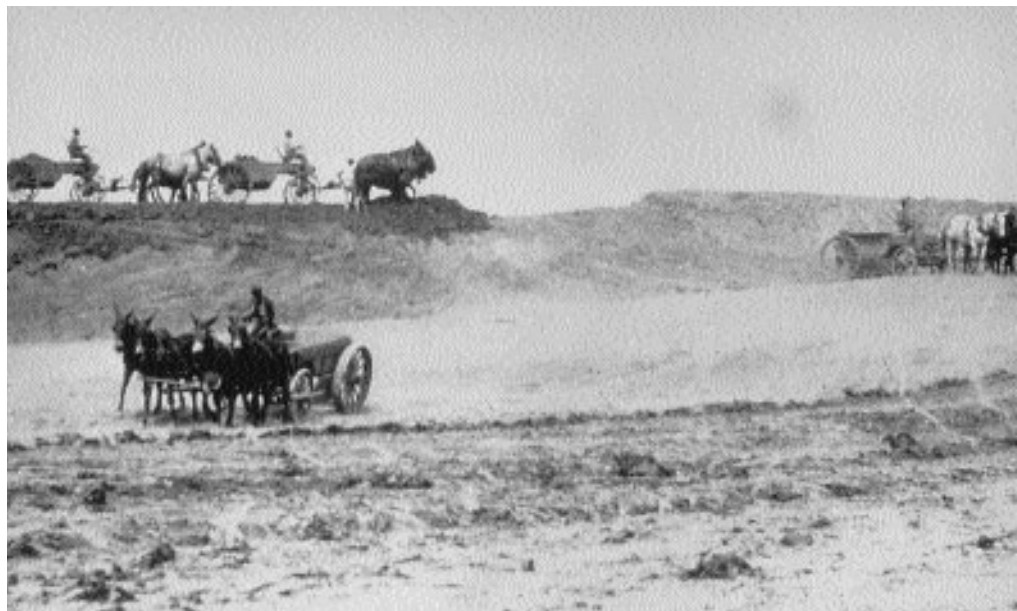
Early levee construction
