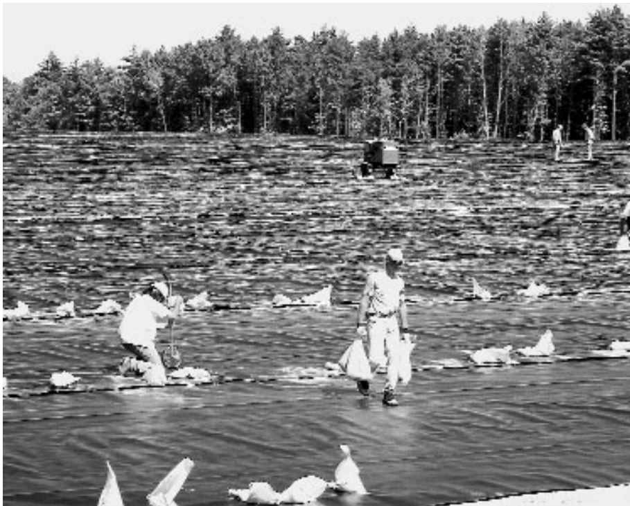
Geo membrane and gas vent layers covering a landfill at K. I. Sawyer Air Force Base, Mich., 1996
