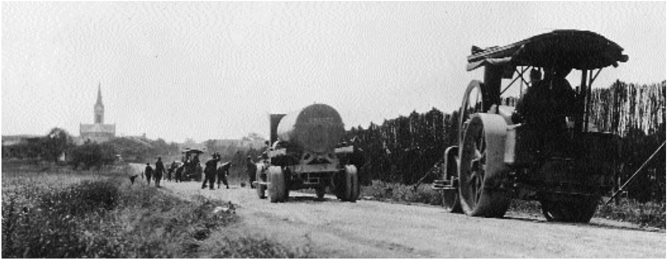
Road construction, France
