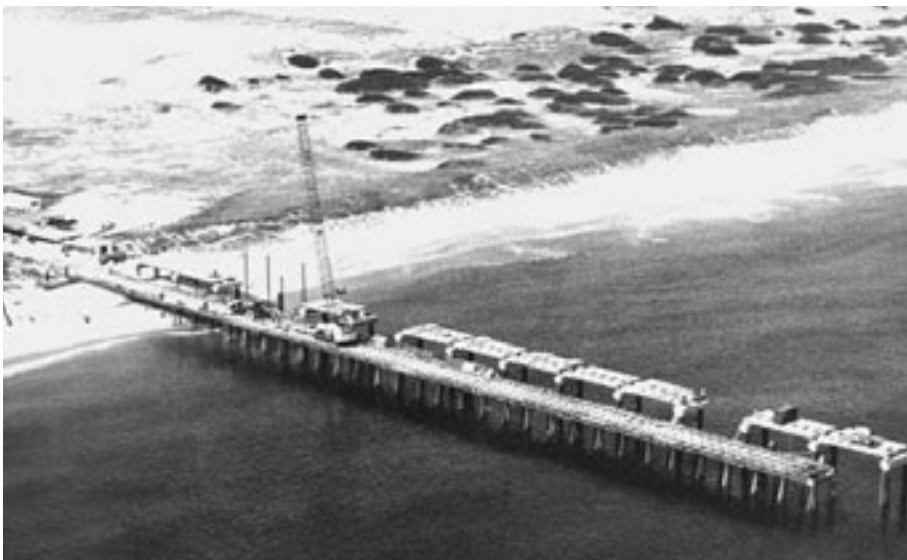
Construction of "the Pier" in the late 1970s at the Field Research Facility, located near Duck on the Outer Banks, N.C. The facility was part of the Coastal Engineering Research Center, established in 1963 to study coastal engineering problems. After several moves and reorganizations, the center became part of the Coastal and Hydraulics Laboratory of the Engineer Research and Development Center.
