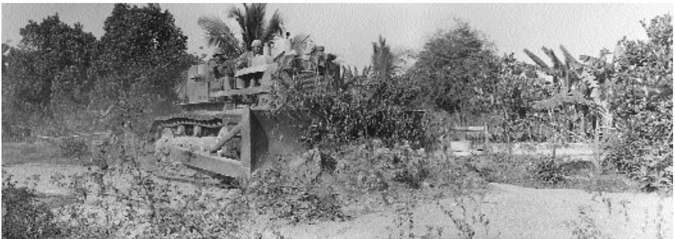
Land clearing at Ben Cat, South Vietnam
