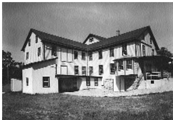
Restored Gruber Wagon Works, Berks County, Pa.
