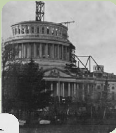
Capitol dome under construction, 1861
