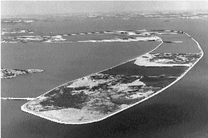
Point Mouillee confined disposal facility, Mich.
