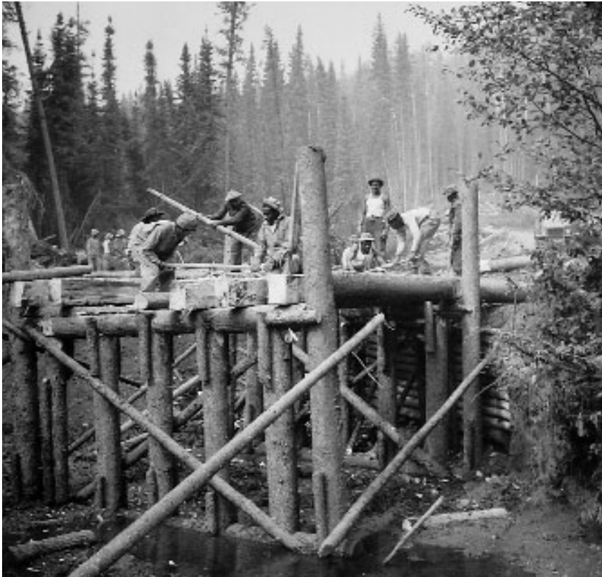
Soldiers of the 95th Engineer General Service Regiment, an African-American unit, building a bridge on the Alaska-Canada (ALCAN) Highway.
