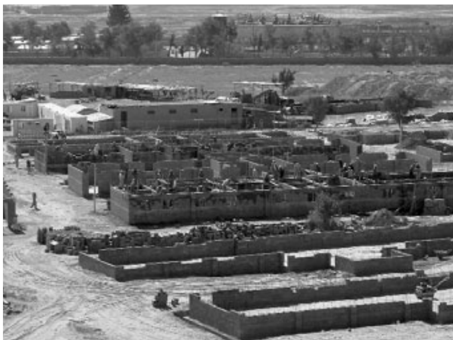
Barracks take shape at the Afghan army's Central Corps headquarters at Pol-e-Charki. Building the army facilities was the first major construction program in Afghanistan in decades, August 2003.
