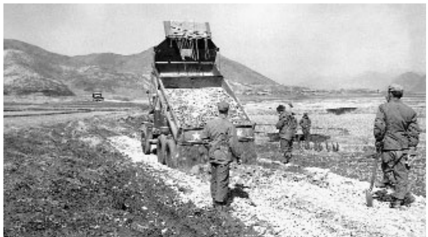
Men of the 65th Combat Engineer Battalion reinforce a muddy road on the north bank of the Han River, March 1951
