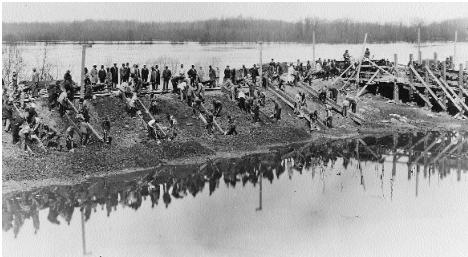
Shoring up a levee near Memphis, Tenn., 1927
