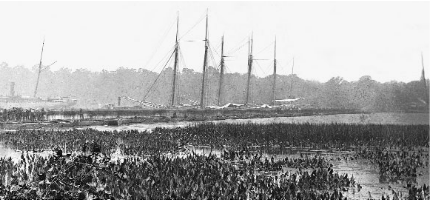
Ponton bridge, held in place by ships, across the James River, June 1864.
