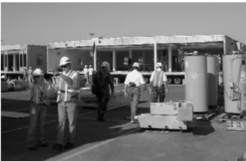
Corps of Engineers personnel supervising the placement of a community health facility in Chalmette, La., October 2005.
