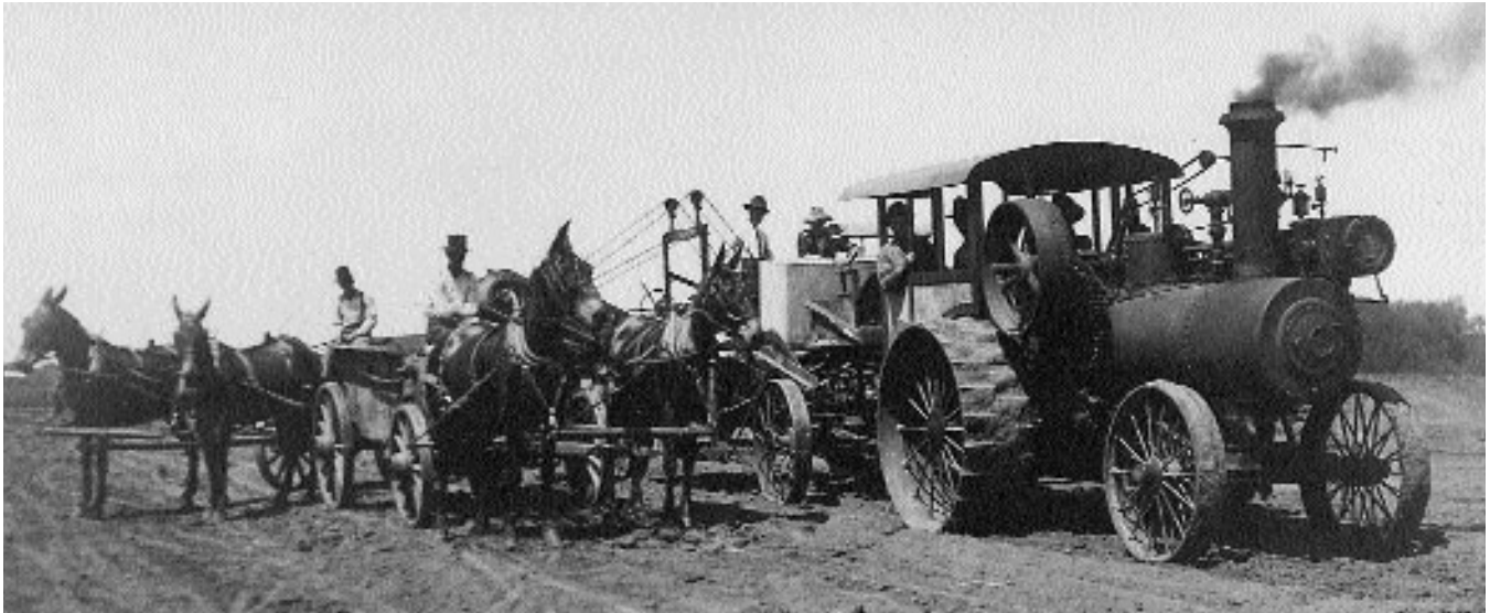
Excavating the Illinois and Mississippi Canal, 1904
