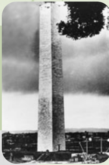
Washington Monument nearing completion, early 1884 National Archives
