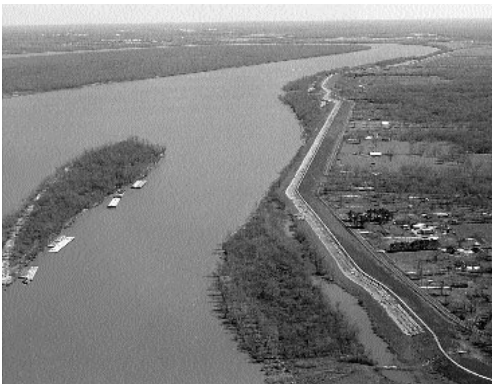
A flood control levee just below Medora Crossing on the Mississippi River at Mile 210
