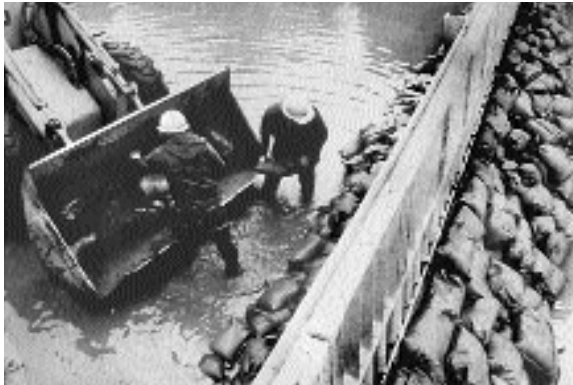
Corps personnel laying down sandbags
