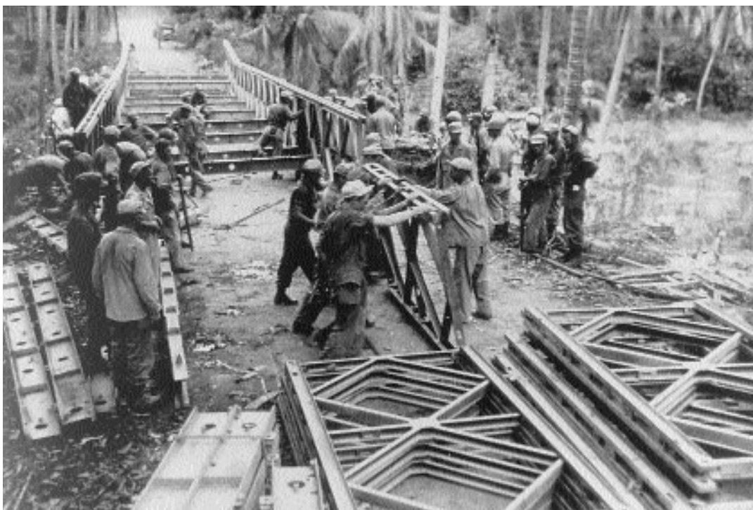
Building a Bailey bridge, the Philippines, 1945
