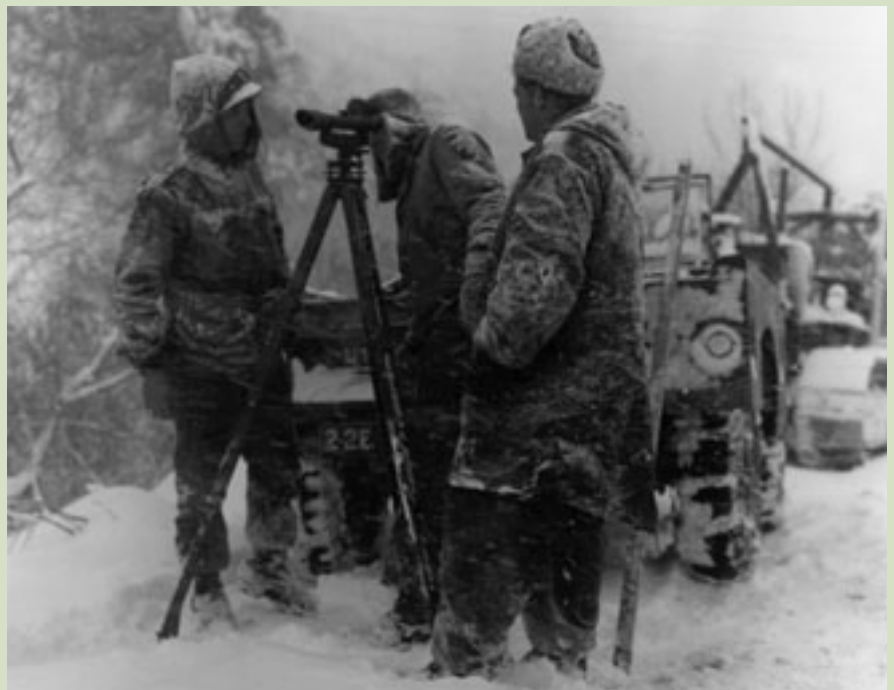
Snow and bitter cold made operations in Korea difficult. Here, soldiers of the 2d Engineer Combat Battalion survey a new supply route.
