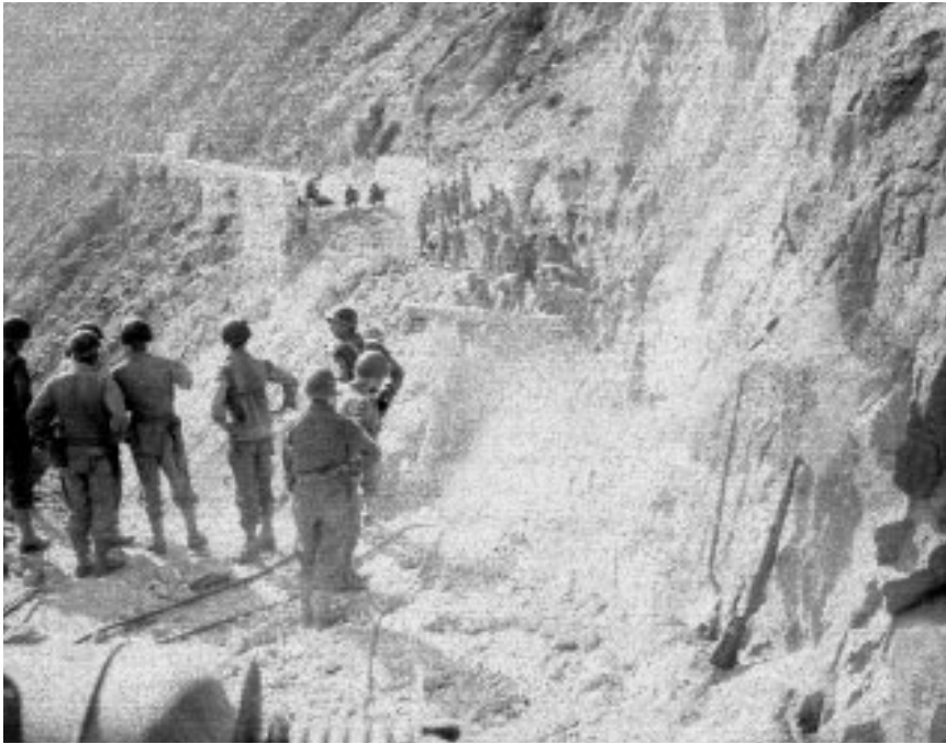
(above) Lacking Bailey bridging equipment, the 10th Engineer Combat Battalion "hung a bridge in the sky" using captured timbers to cross this gap in the road at Cape Calava, Sicily, August 1943.
